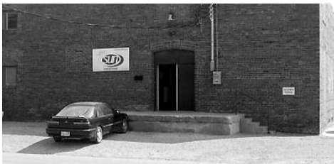
Above: c. 1950 photograph of masonry openings and concrete docks, Barteldes Seed Company. Below: Current condition of the same entrance.
