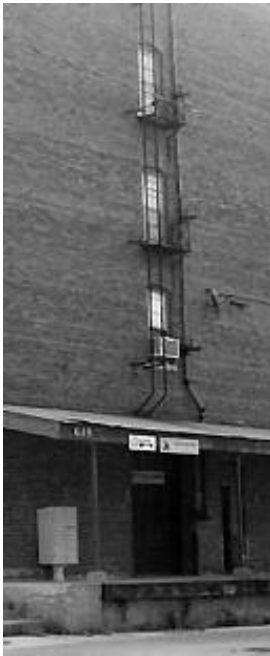
Existing metal features – Zone 1
