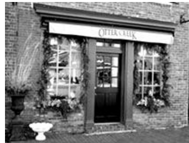
The infill storefront in the building above creates the false impression of an original retail store rather than the historical industrial use of the building
