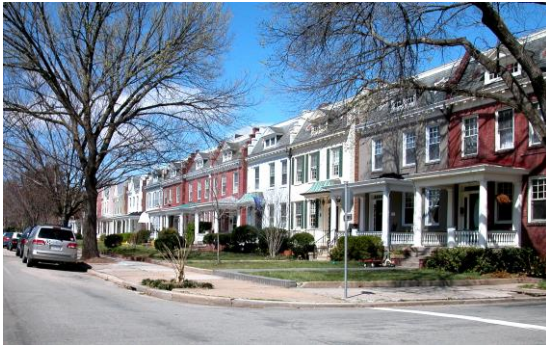
Example of Housing Density and Fenestration
