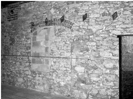
Existing brick and stone masonry – Zone 1
