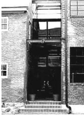
This small glass connector between two historic buildings is appropriately set back. A similar approach may also be made between a historic building and an addition
