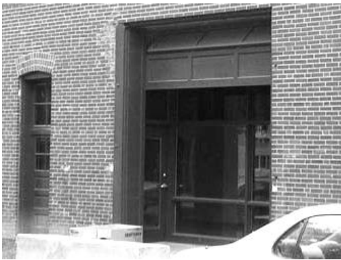
Original door opening is retained. The new infill incorporates an entrance and half “closed” garage door as well as transparent glazing is an appropriate treatment where there is no documentation of the original door.
