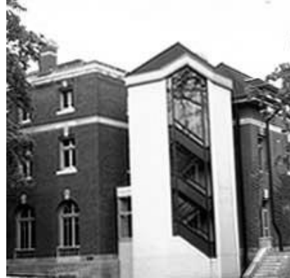
Stair tower could have been incorporated in the building by enclosing existing stair well. Location of the new stairwell on a highly visible façade is inappropriate as is use of materials and scale and massing
