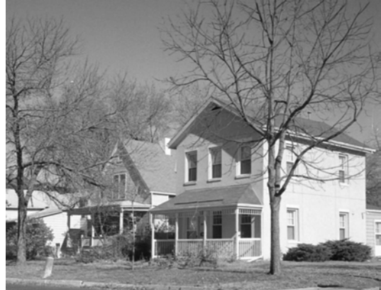
These structures are good examples of appropriate windows and doors because of their vertical proportions.
