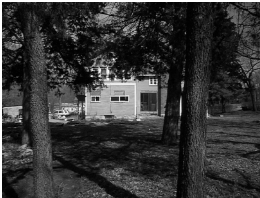
The new horizontal windows are an inappropriate response to the character of the existing house and surrounding structures.
