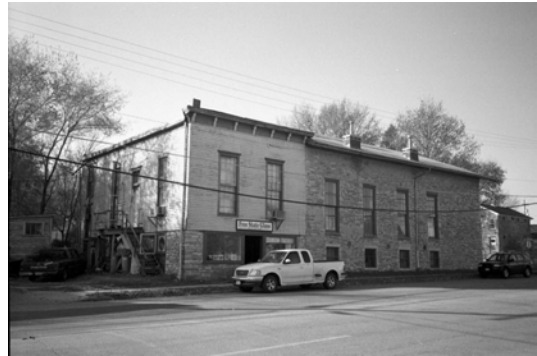
Many of the older commercial structures have flat roofs with a parapet along the perimeter. New business structures should respect these roof patterns.
