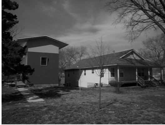
Both of these structures are inappropriate response to “ Roof Shape ” because the roof pitch is too flat.
