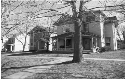
While maintaining appropriate scale and massing, the structure on the left is an inappropriate response to “ Building Masses and Spaces ” because it is setback further from the street than adjoining structures.
